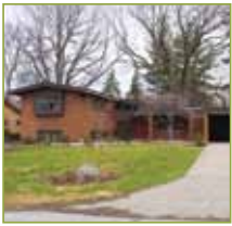
1. Edward Hertel Residence 1631 Walnut Hills Drive Manson & Jackson, 1958
